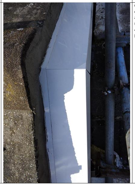
Gable apex: Preformed apex flashing with cover strip over. Cover strip extends into space between roof tiles and apex flashing & rendered in with flexible, polymer-modified cementitious filler.
