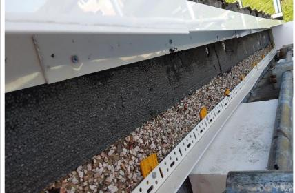
20 mm EPS-Premium insulation ( $\lambda 0.030$  W/mK; R > 0.6 m<sup>2</sup>K/W) incorporated between roof closure profiles and substrate. Extends from eaves to apex along full length of gable.
